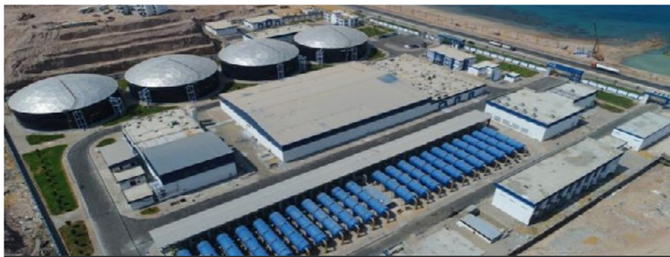
Fig. 5. El-Galalah (RO) Water desalination plant [33].
