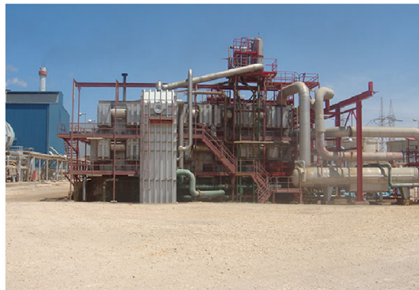
Fig. 2. Multistage flash desalination plant at Ayoun Mosa, Egypt [29].
