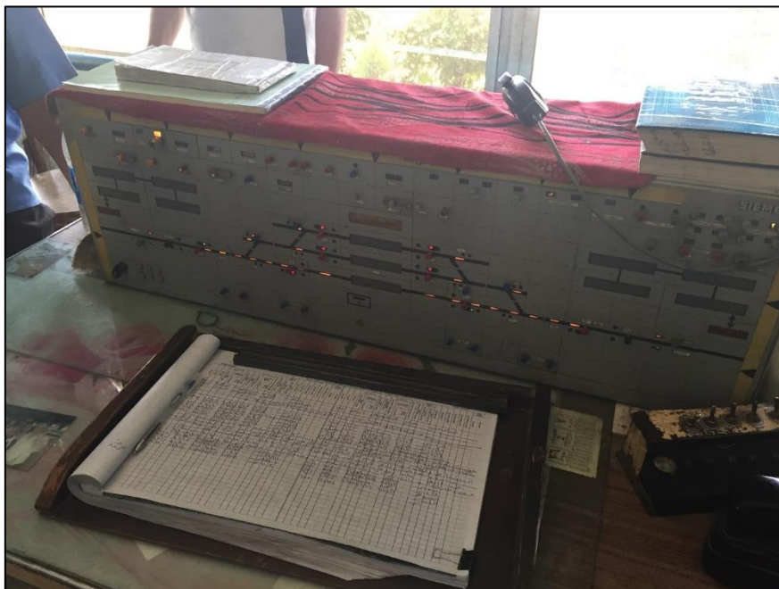
Figure 14 – train control equipment at Ataa station Source: Site visit
