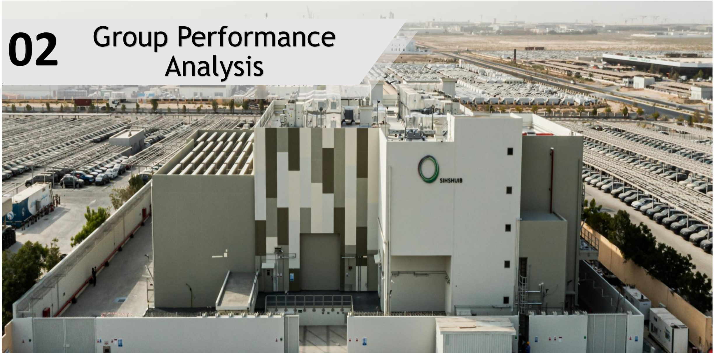
132/11 kV SIHSHUIB Substation – DEWA (UAE)
